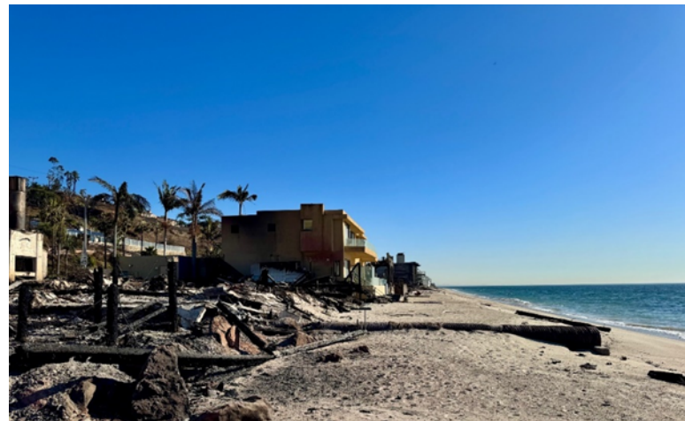
Figure 2: The Palisades Fire burned to the beach, taking many homes along the coast in its path. Some of the surviving buildings illustrated effective home hardening, such as having dual-paned tempered glass windows.
