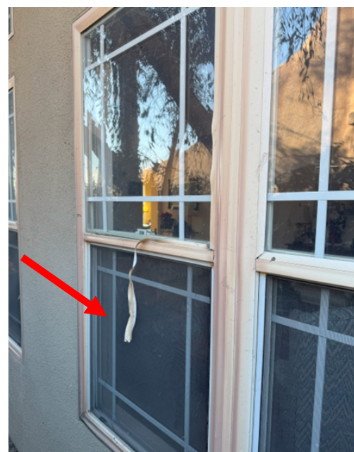
Figure 6: Radiant heat damaged this window. Note the vinyl glazing is deformed. In some cases radiant heat led to window panes breaking or falling from the frame.
